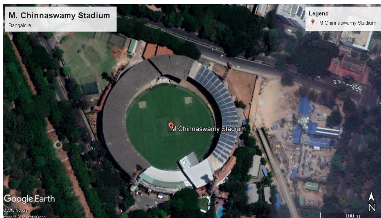
Figure 2-6 Google Earth image of the Solar PV plant set up at M. Chinnaswamy Stadium, Bangalore
