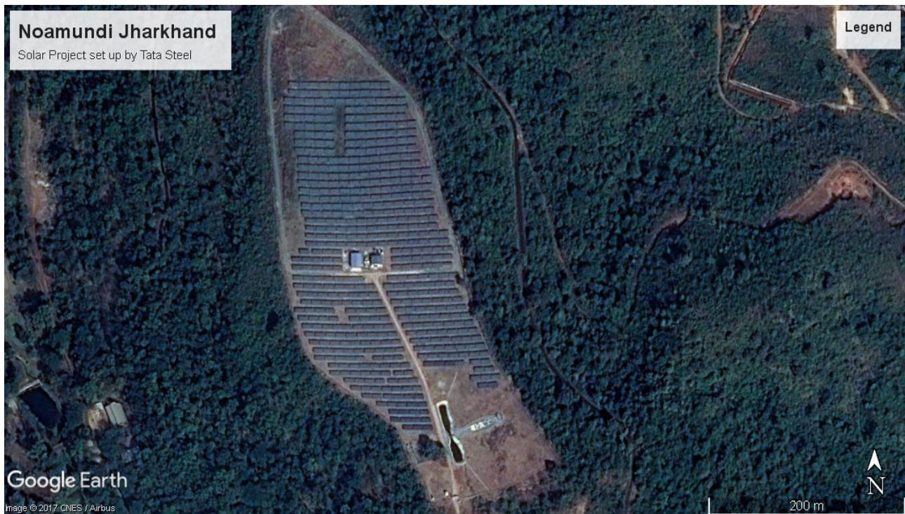
Figure 2-5 Google Earth Image of the Solar PV plant set up at the iron ore mine at Noamundi, Jharkhand
