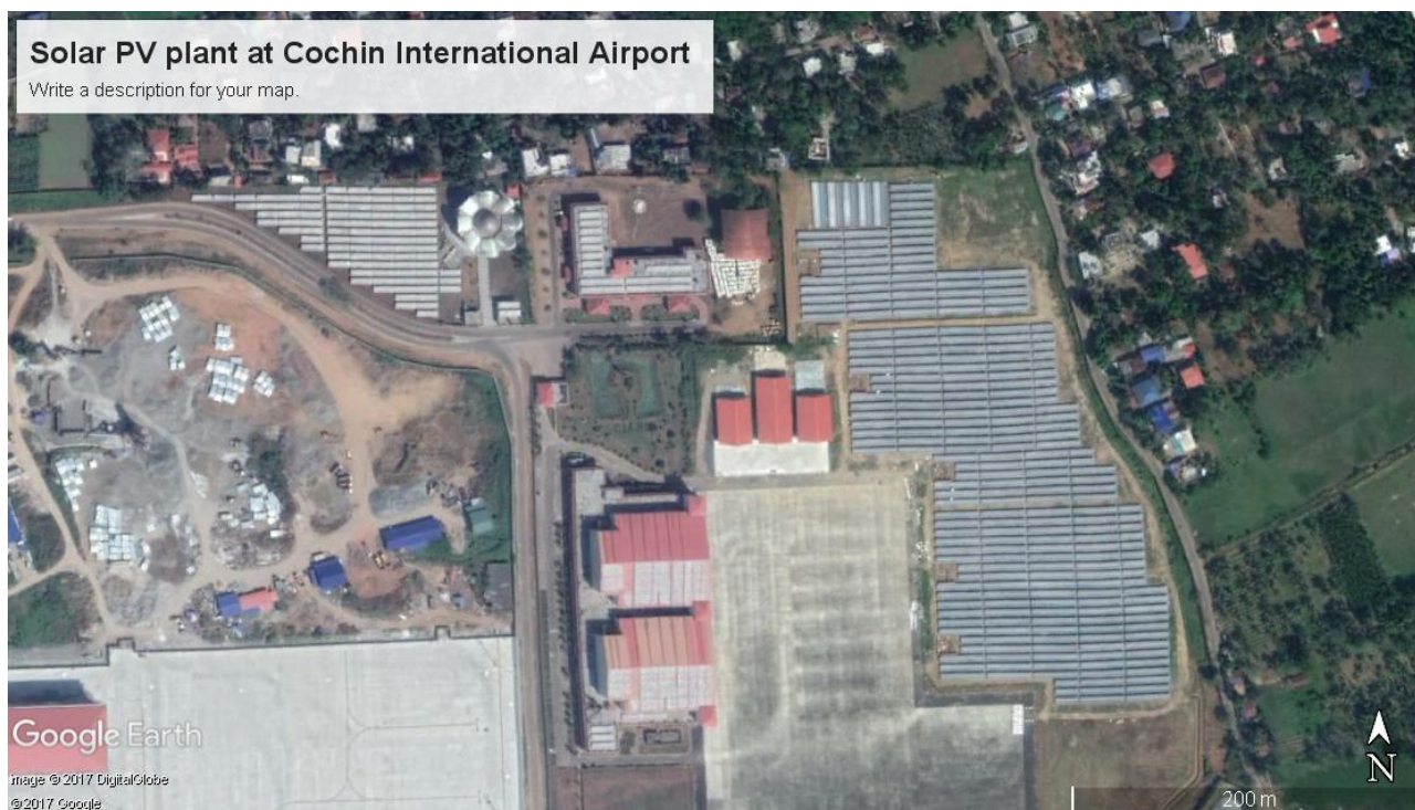
Figure 2-7 Google Earth image of the Solar PV plant set up at Cochin International Airport
