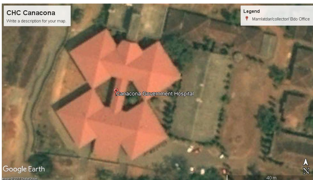
Figure 3-5 Google Earth image of selected Govt. building
