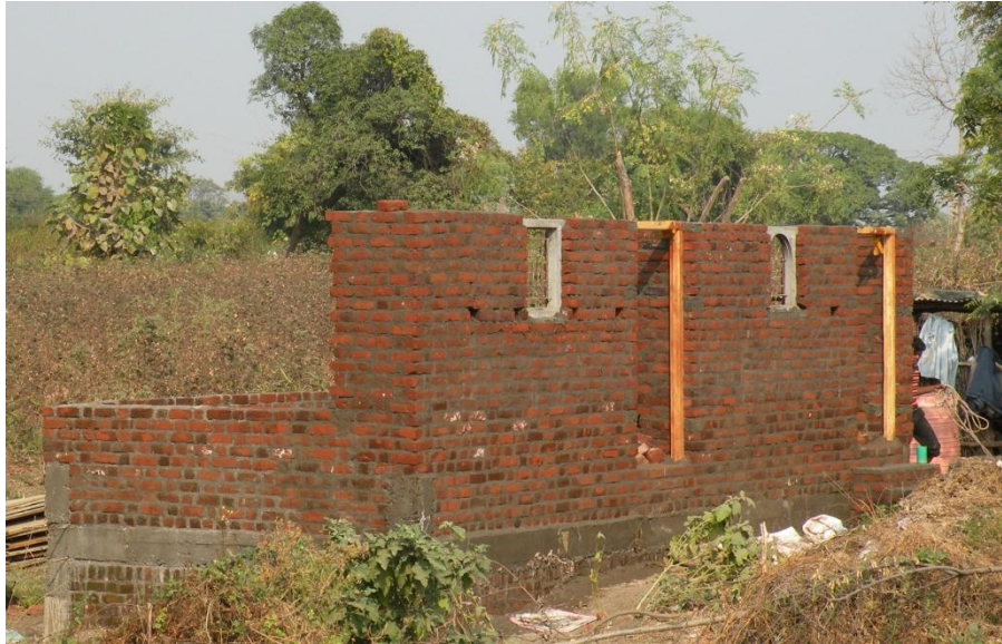
Figure 2.2: House construction going on under the IAY
