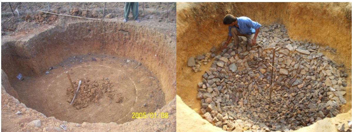
Figure 4.4: (a) Digging of pit for FDBP (b) Arranging stones for base
