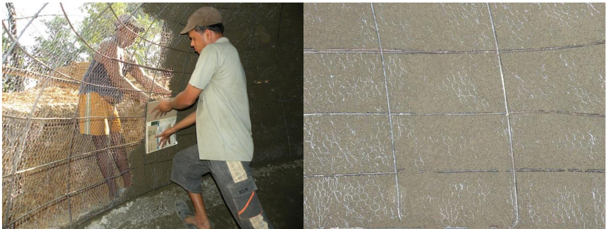
Figure 4.3: (a) First layer of concrete of FDBP (b) Concrete latched to chicken mesh
