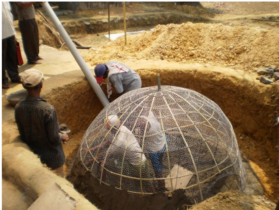
Figure 4.7: Constructing dome with Bamboo frame
