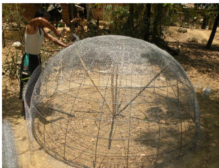
Figure 4.2: Steel cage of the FDBP dome
